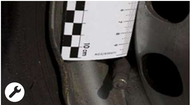
On steel rim: Attachment edge slightly deformed
