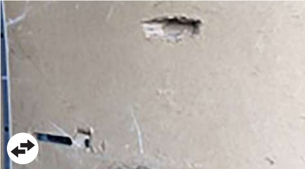
Wood internal protections: Impacts, torn panel, panel missing (excluding door upper panels)
